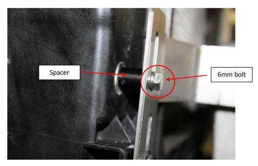
10. Using a 10mm socket tighten both bolts installed in step 8 and 9.
